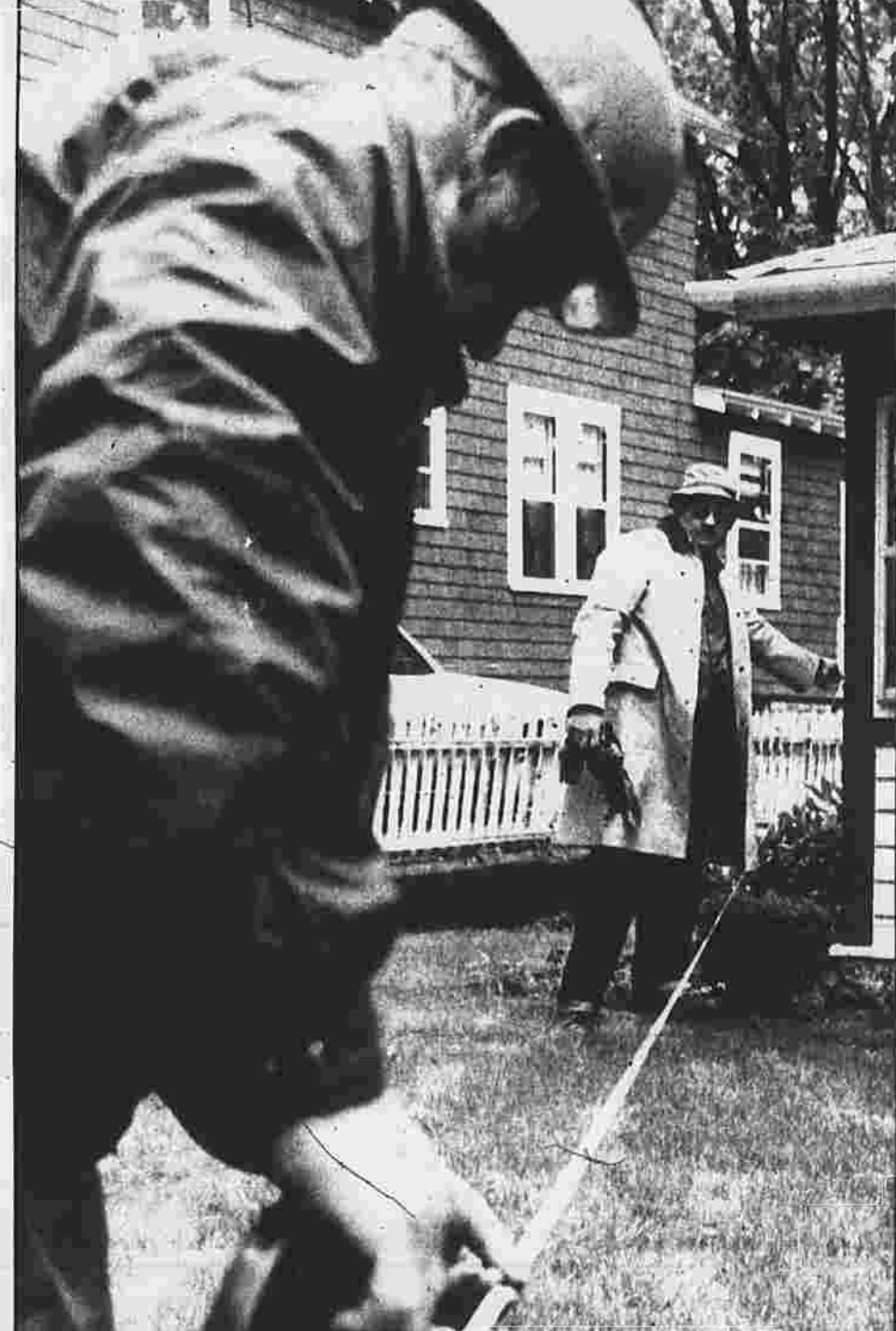
On a reeled curb box at a home on Summit Street this morning, the two employees of the Manchester Water Department were shutting off service and took new measurements in case they needed to locate the box again to restore water to the home.
